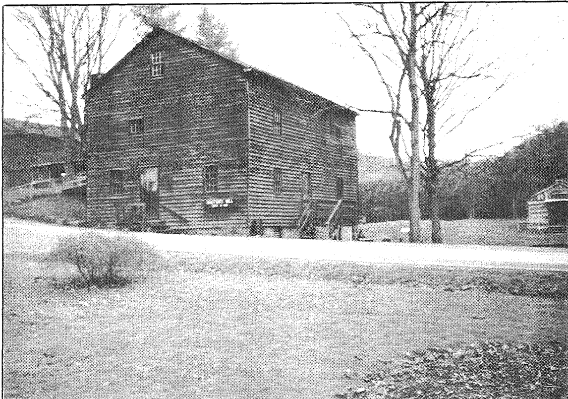
Gaston's Mill, restored and operational. Flour is ground on weekends at the mill built in 1835.
