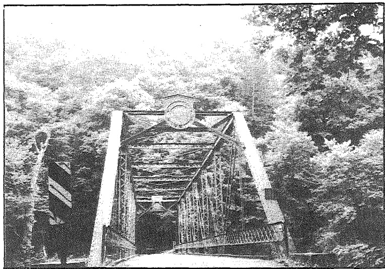
The Columbiana county highway department bridge 1025 over the Little Beaver Creek erected in 1910.
