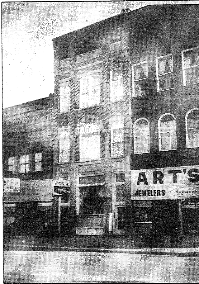
The Ohio Mutual Insurance building, constructed in 1876, and occupied today by Recreation Billiards.
