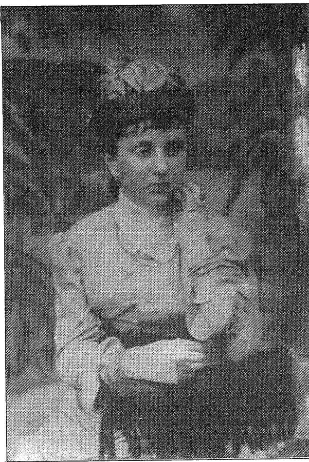
Sade Emmerling, 25, is shown in this formal photograph taken about the time of the Scioto excursion trip. Sade was drowned along with her husband, Mike. Both were East Liverpool residents.
