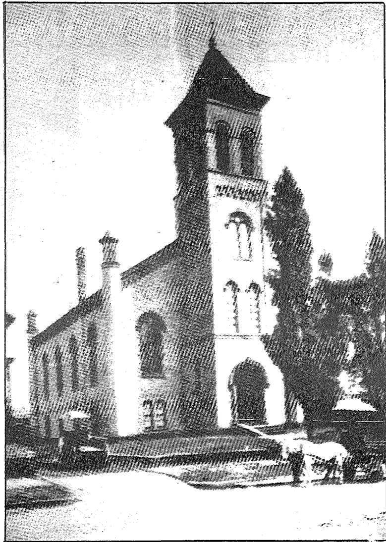
Salem Methodists built this handsome brick church along Ellsworth Avenue in 1859. The congregation was known then as the First Methodist Episcopal Church; that was changed in 1939 with the merger of the Methodist Episcopal, Methodist Episcopal South and Methodist Protestant.
