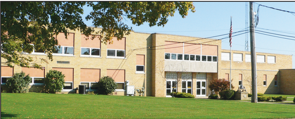
Shown is the exterior of Greenford Bobcats Space Center. (Salem News photo by Kevin Howell)
