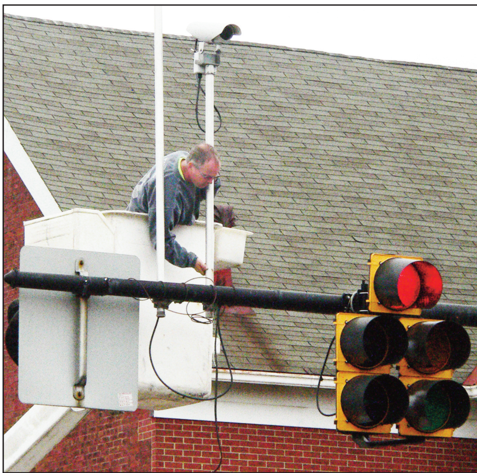
Salem city electrician Mike Bibbee attaches a sensor to the traffic light fixture at East State Street and Lincoln Avenue Tuesday morning, finishing up replacement of the pole on the southeast corner. (Salem News photo by Kevin Howell)
